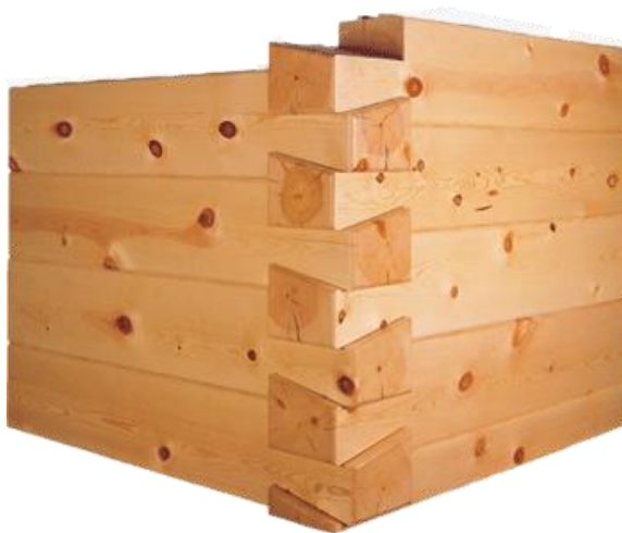
Picture: 1.78. Through Dovetail
